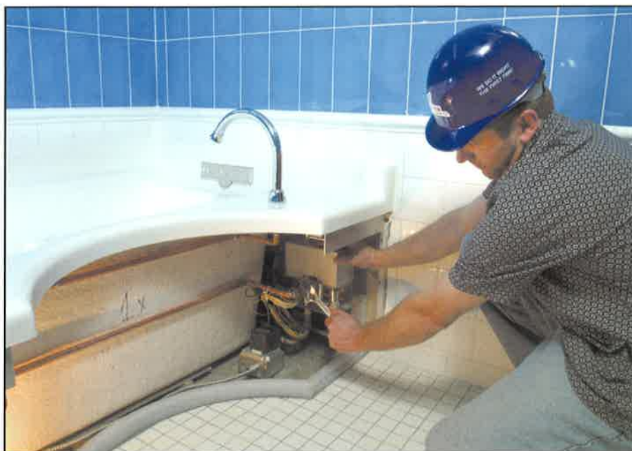
Custom-designed TAG Tubs were installed at the Broadmoor, with minimal effect on existing tile surfaces.
